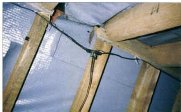
Fig. 3: Photo showing the centre feeder connection of the h.f. antenna. The conductor is supported to the timbers by a cord, while the helices are wound on roof timbers insulated by a plastic membrane (but large diameter plastic piping could be used as an alternative).
