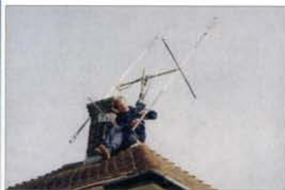
Fig. 2: The reflector assembly being fixed to the end of the boom.
