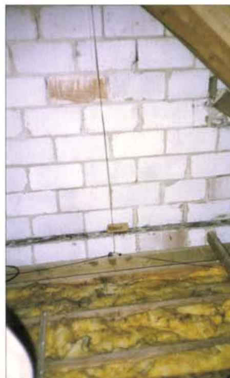
Fig. 2: An L-type dipole located at the opposite gable end cut for the 29MHz band. This has a very low v.s.w.r. and is useful for 28MHz f.m. activities, especially during Es propagation.
