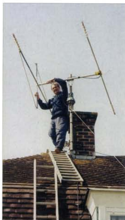
Fig. 4: Peter G3LDO says: "Note the crawling ladders used for mounting the antenna ... don't even think about going on to a roof without these!"
