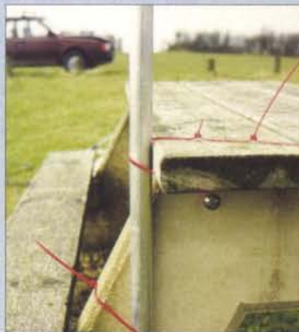
Fig. 1: Colin Redwood G6MXL uses re-usable cable ties to fix the mast to the fence posts, picnic tables, railings, etc. An idea that you might like to try.
